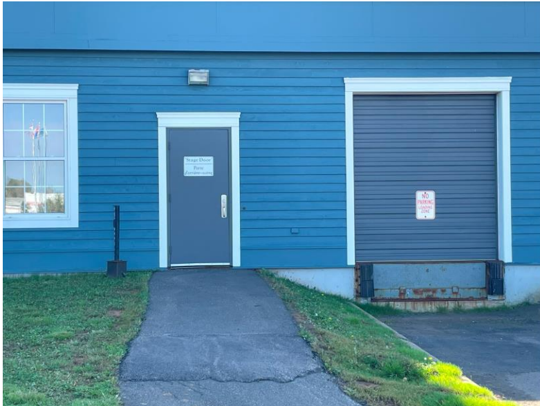
Stage Door & loading dock
